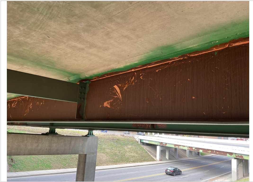
Span 3 Girder C corrosion
