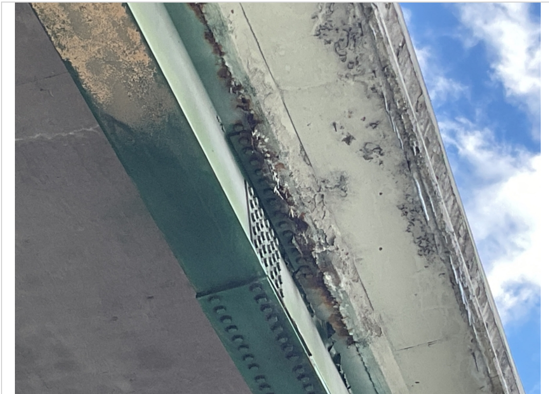
Span 2 Girder A top flange corrosion with eff
