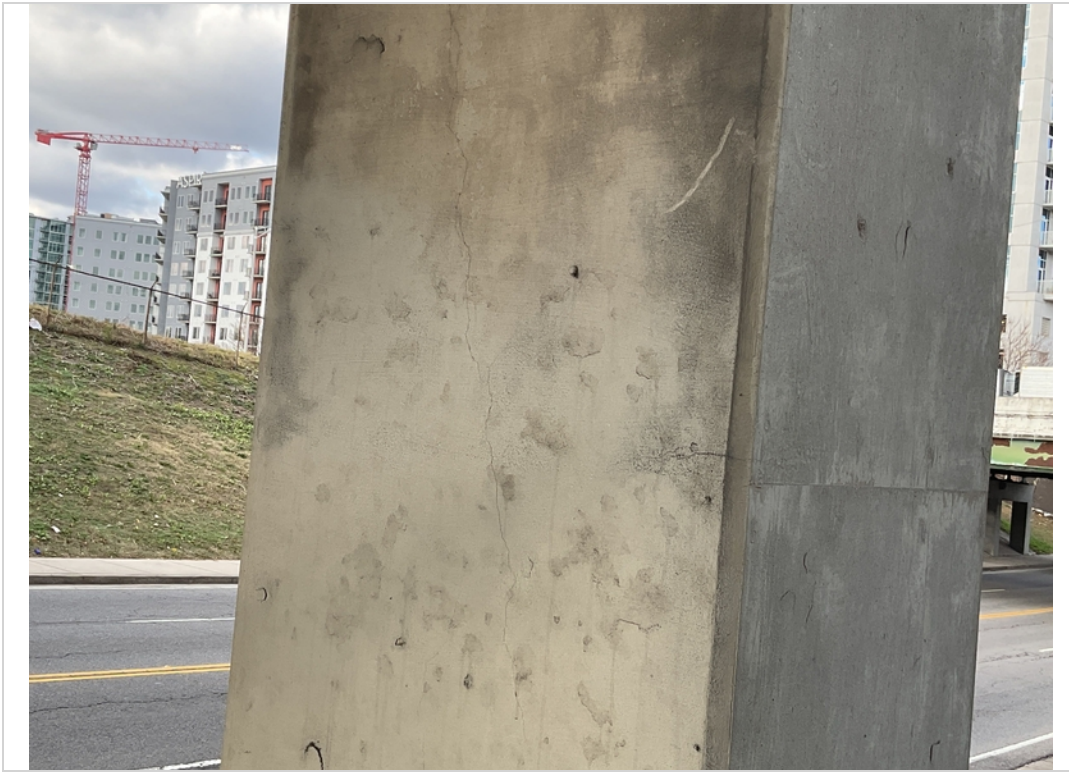
Bent 2 column A vertical crack
