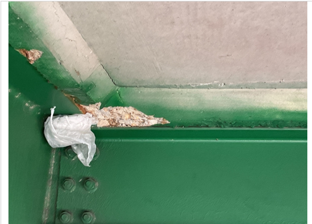
Span 3 bay B spall at abutment 2
