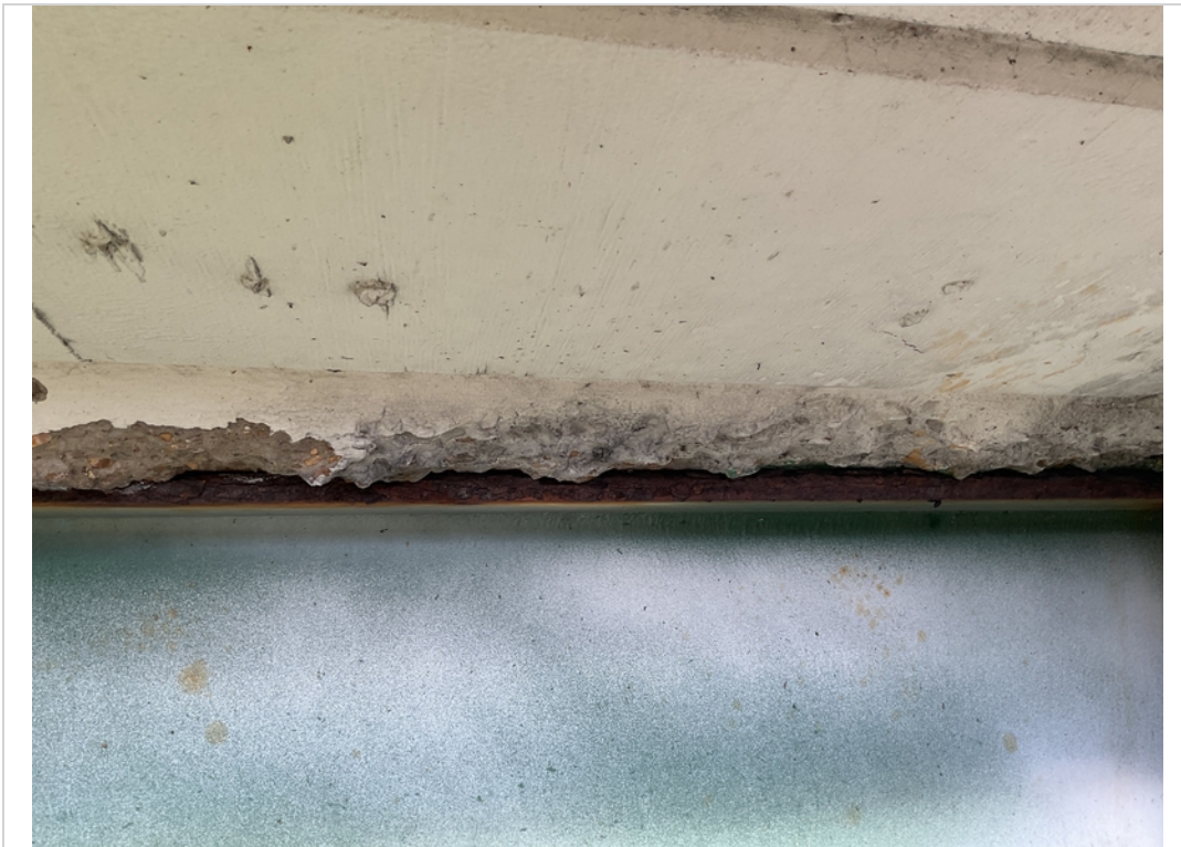
Overhang span 3 right side spall
