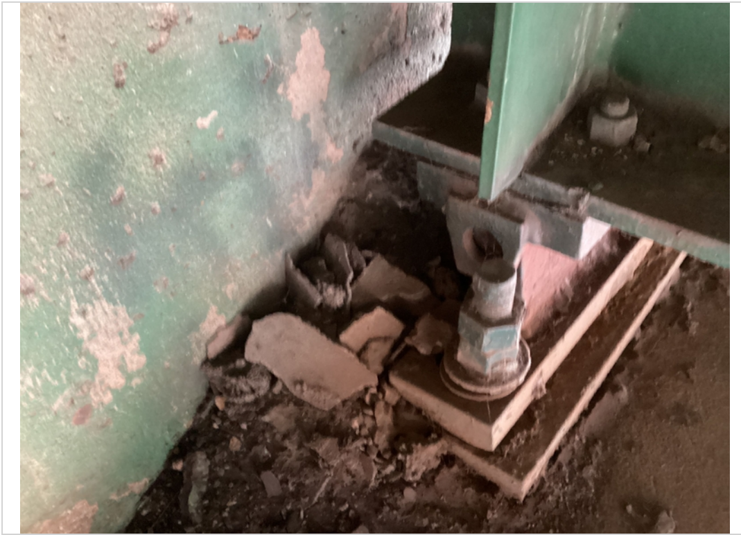
Abutment 1 bearing D missing pin
