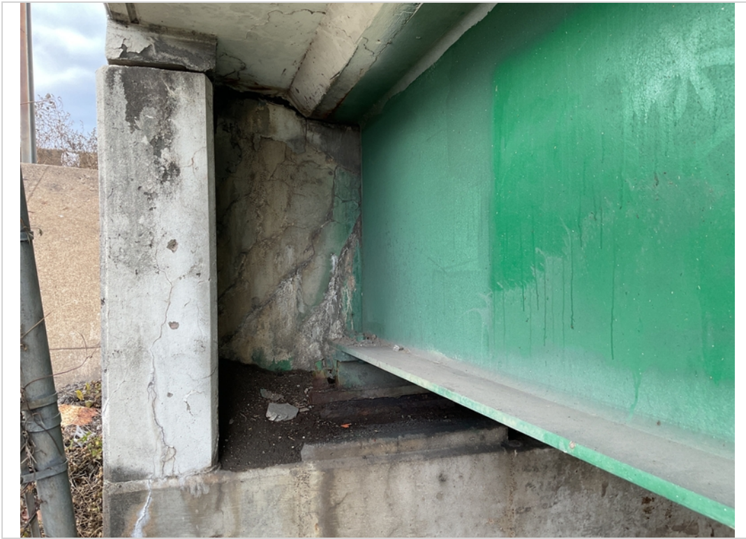
Abutment 1 back wall map cracks with eff
