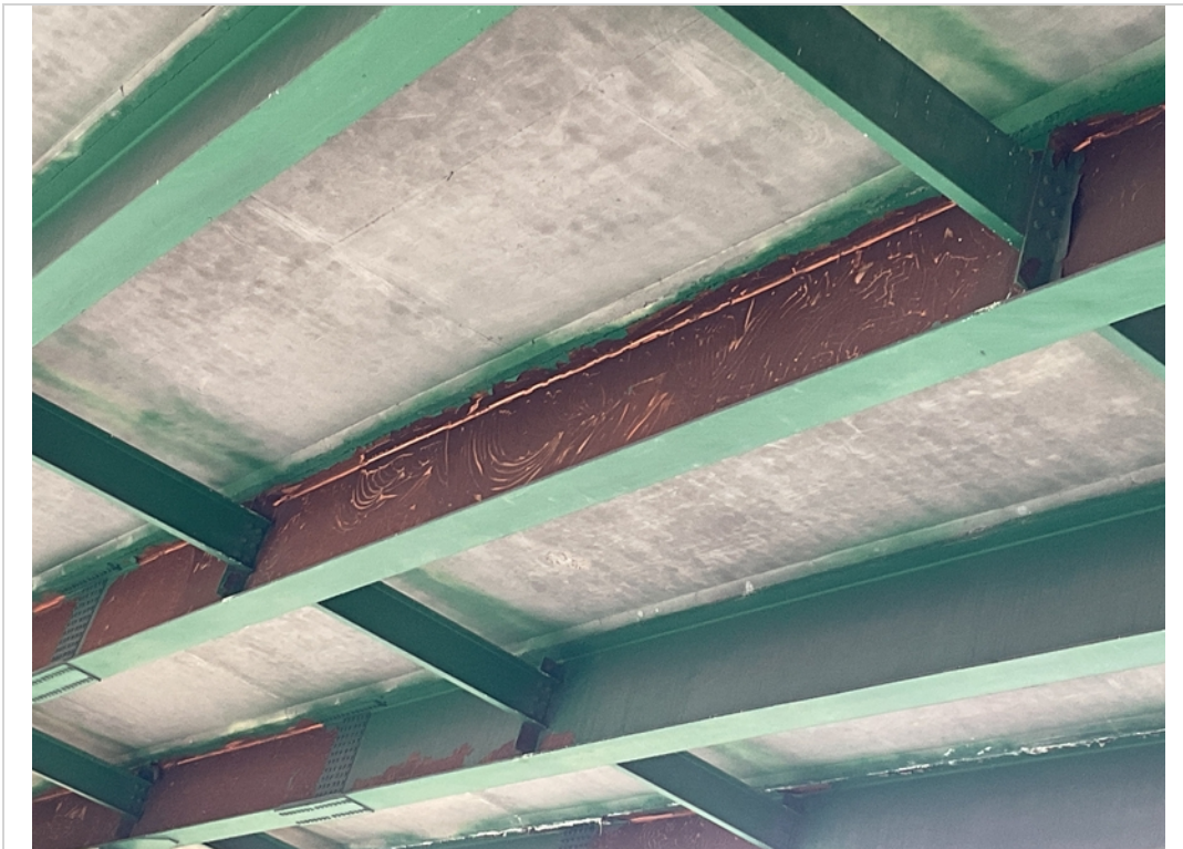
Span 2 Girder C corrosion
