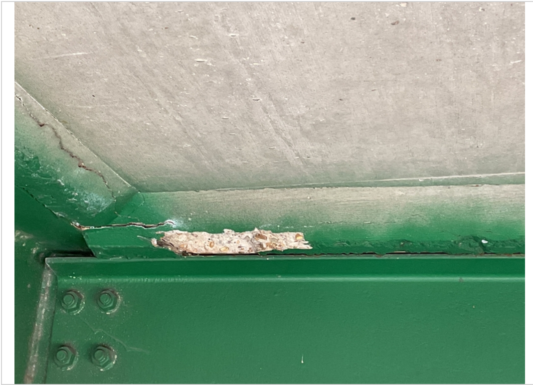
Span 3 bay A spall at abutment 2
