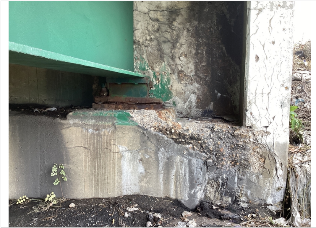
Abutment 1 cap and backwall scale map cracks
