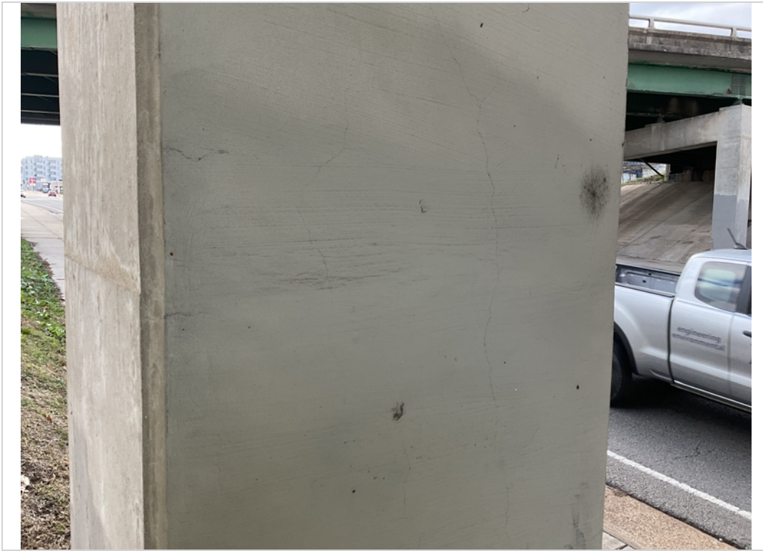
Bent 2 column C vertical crack
