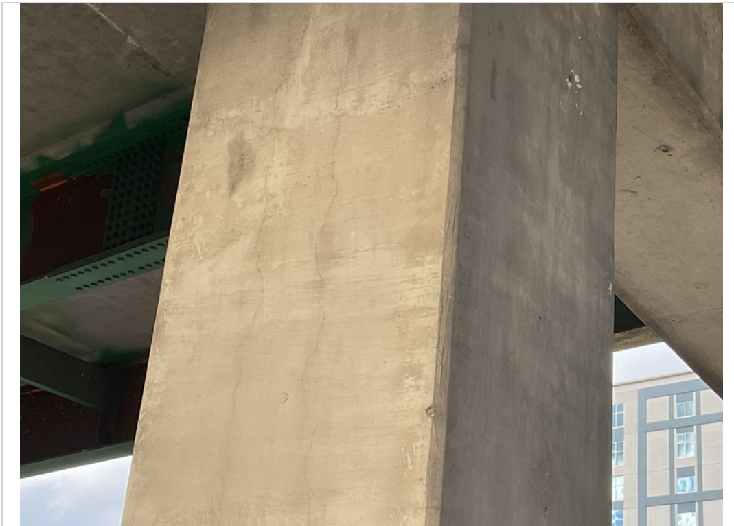
Bent 2 column B vertical crack
