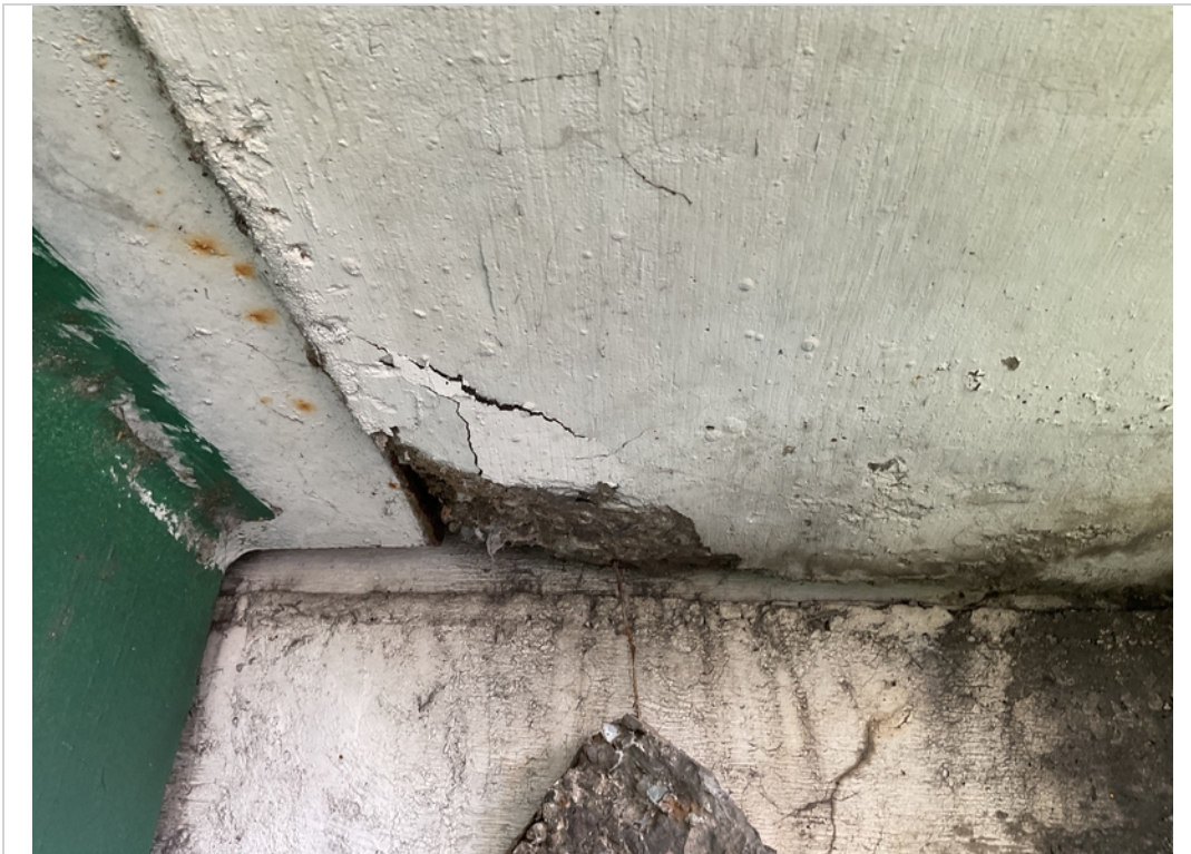
Overhang span 1 left side spall
