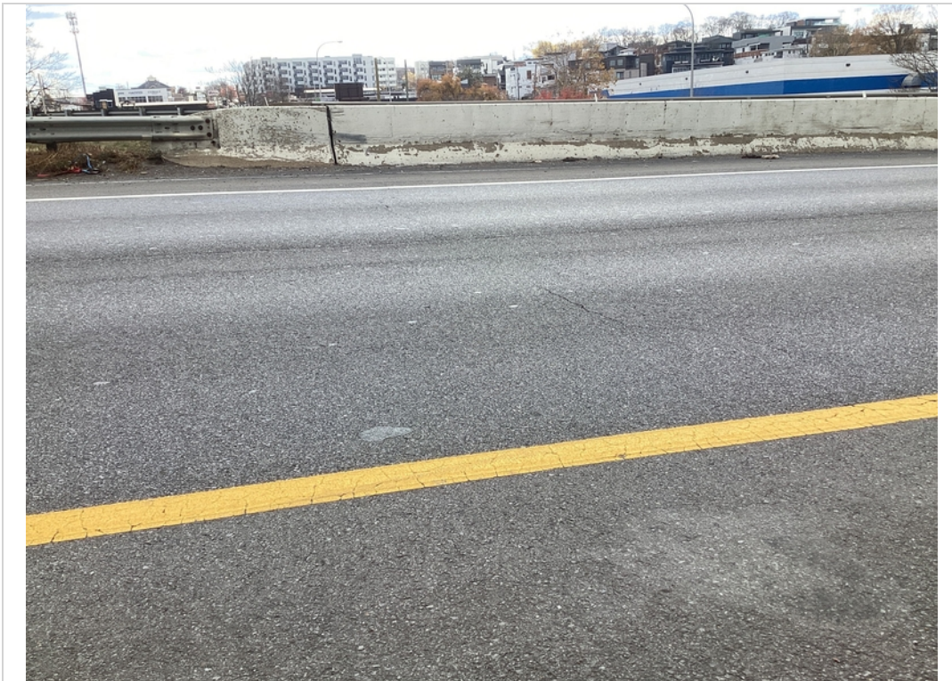
Span 3 transverse cracks
