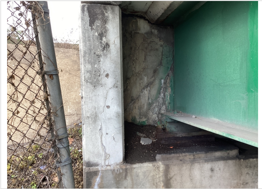
Abutment 1 backwall cracks with eff
