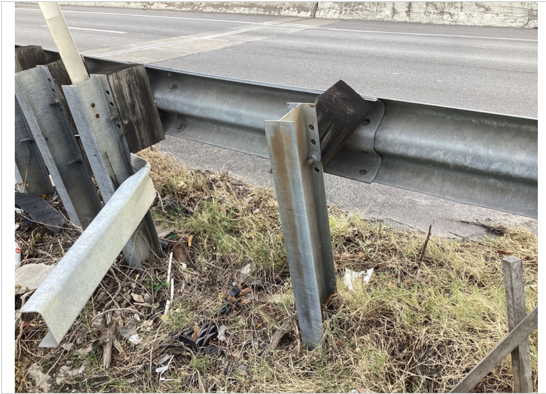
A approach guardrail impact damage
