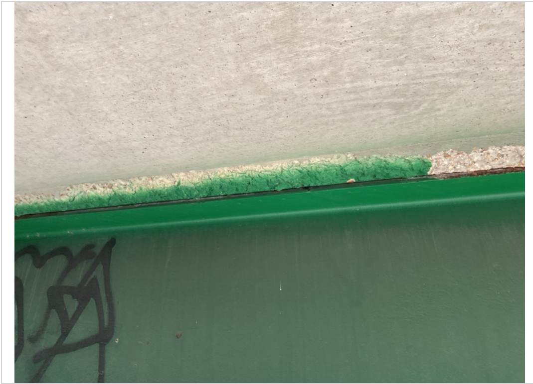
Span 3 bay D spall top flange beam E
