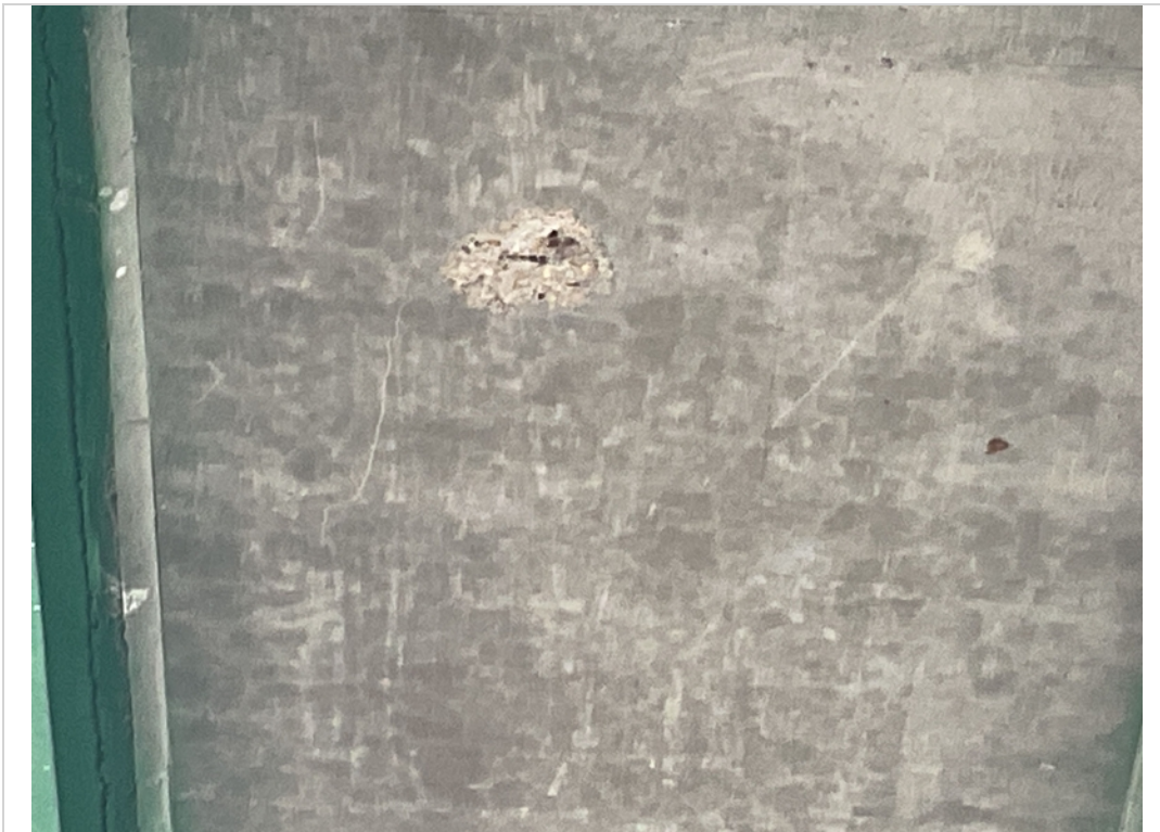
Span 2 bay C spall with exp steel
