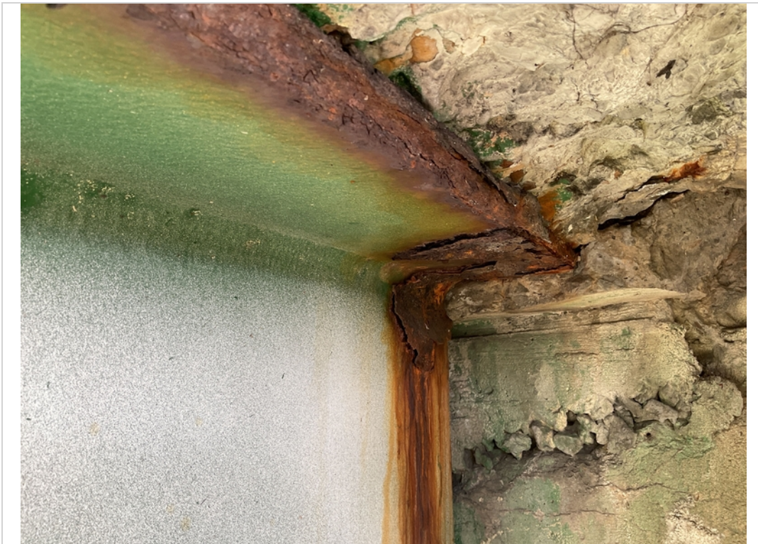
Span 3 Girder E top flange corrosion
