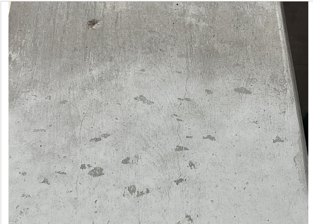
Bent 1 column C vertical crack
