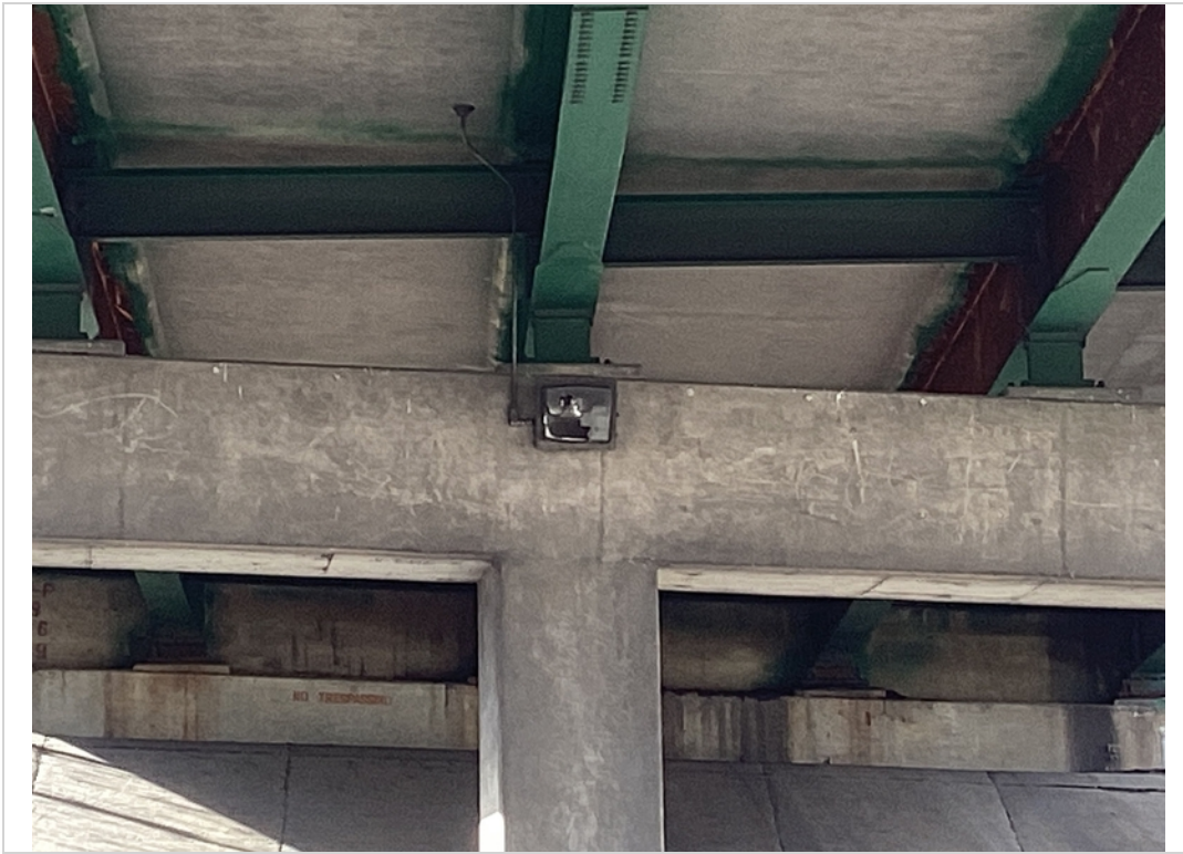
Bent 1 broken light case
