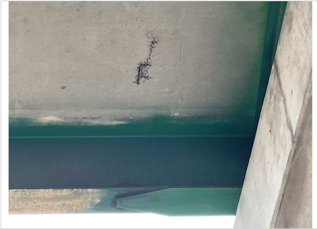
Span 2 bay A spall with exp steel
