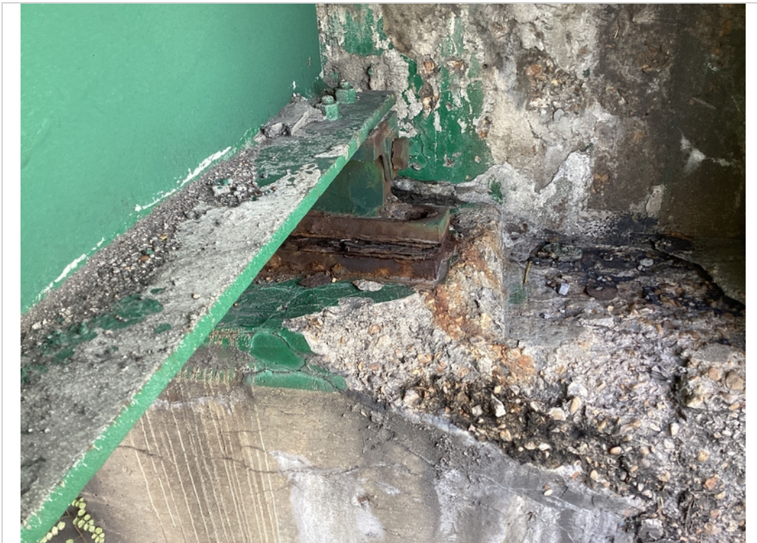
Abutment 1 missing anchor bolt bearing A riser A heavy scale
