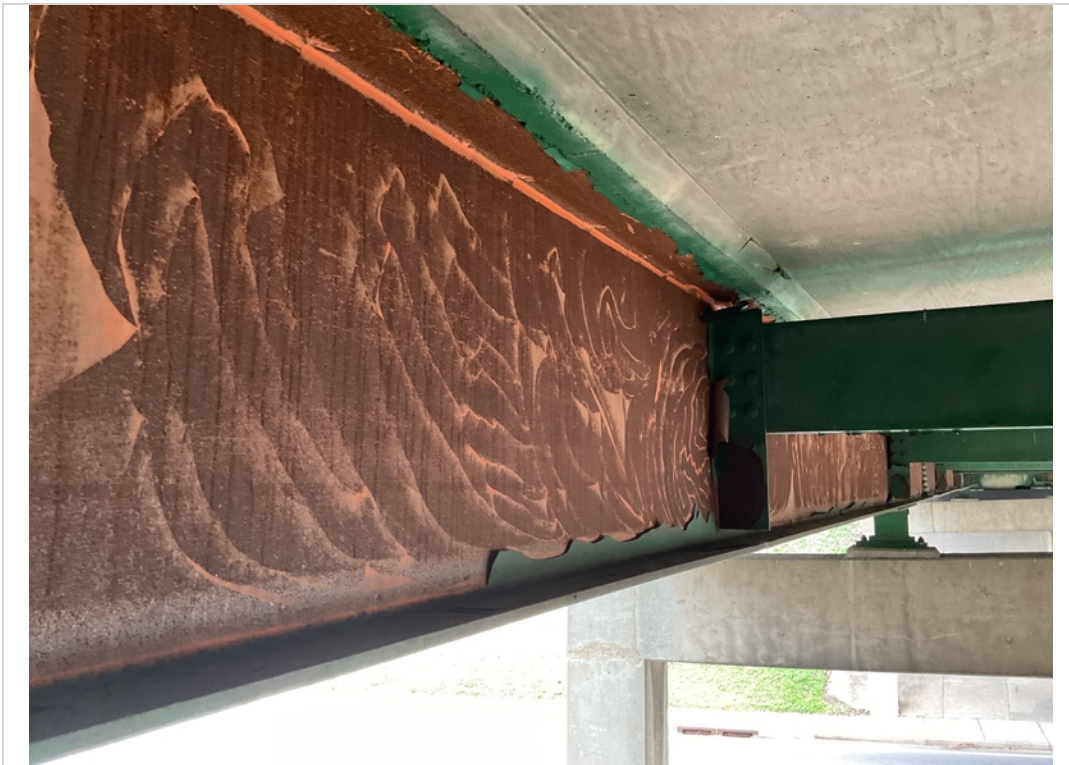
Span 1 Girder B corrosion
