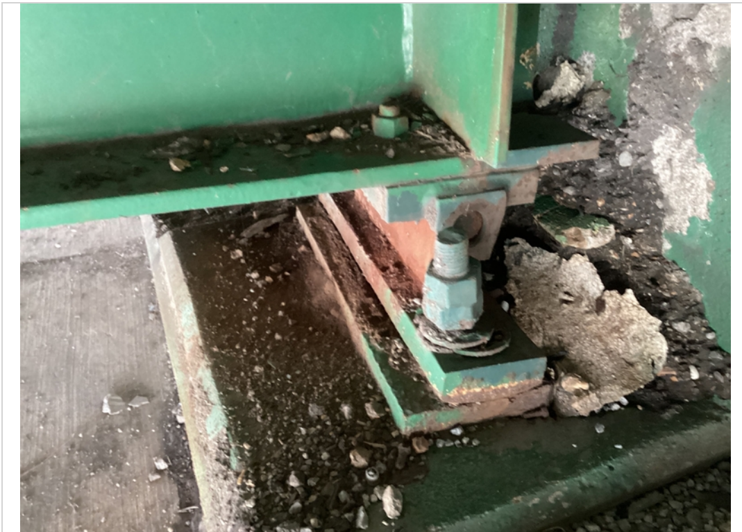
Abutment 1 bearing C missing pin
