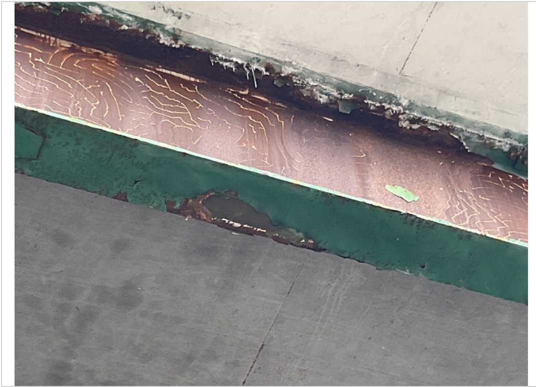
Span 2 Girder E bottom flange corrosion
