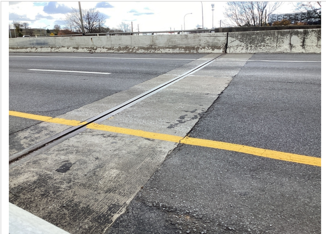
Span 1 joint
