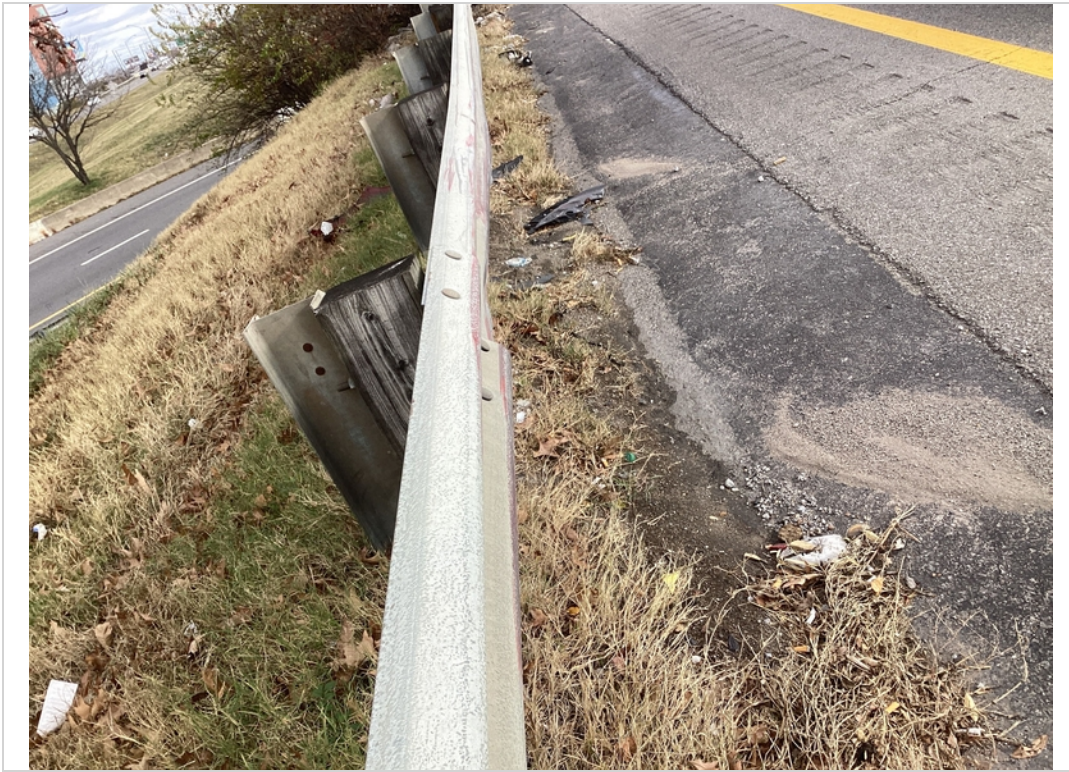
B approach guardrail impact damage
