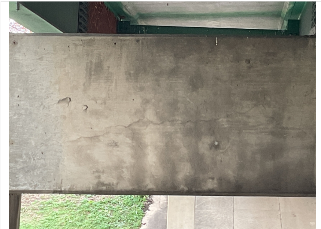
Bent 1 cap horizontal crack
