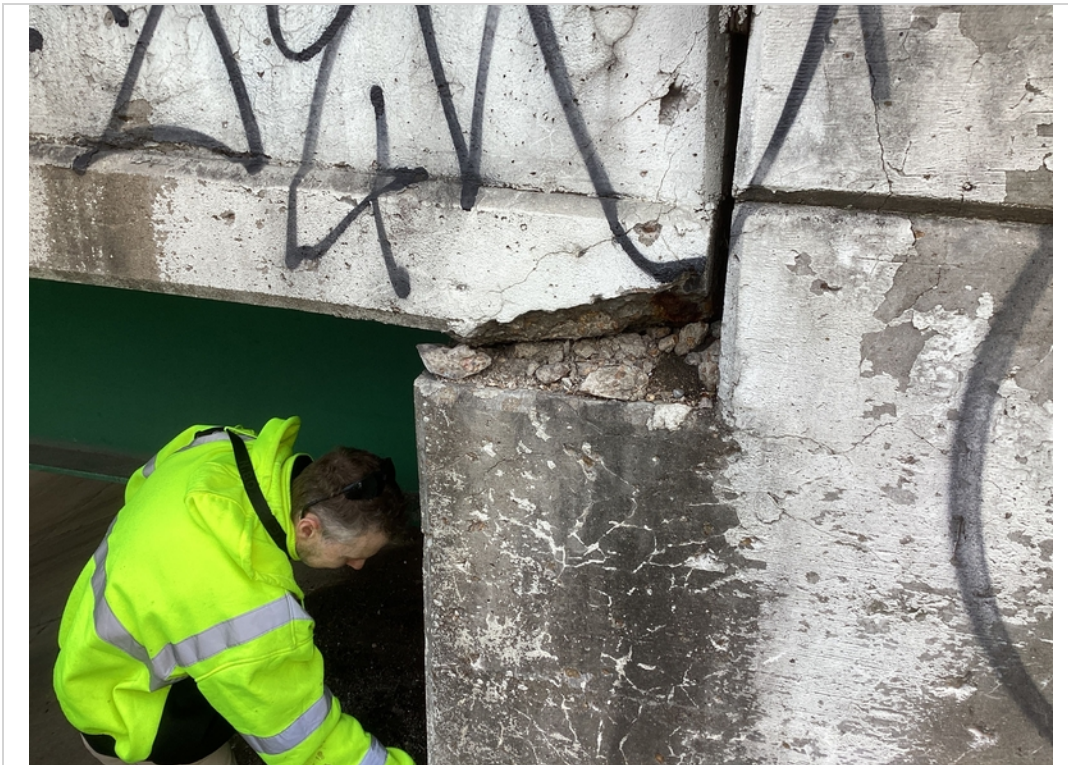
A approach bridge rail spall left
