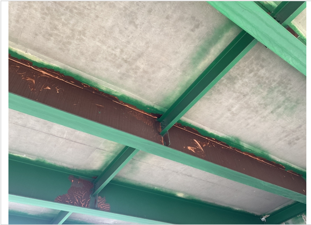
Span 3 Girder C corrosion
