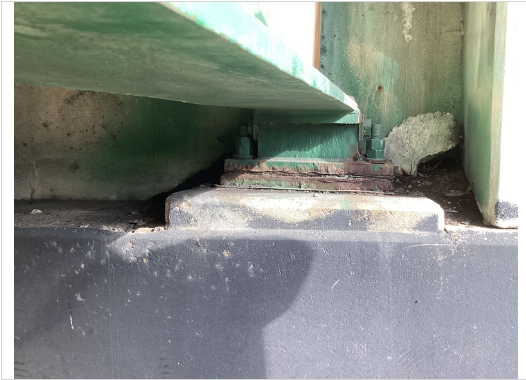
Abutment 2 bearing E light corrosion
