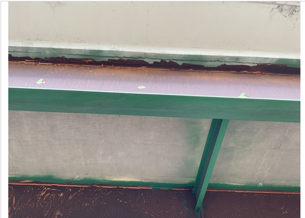
Span 3 Girder E corrosion
