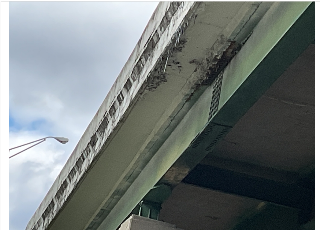
Overhang span 2 map cracks with eff left side
