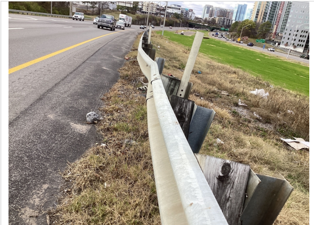
A approach guardrail impact damage
