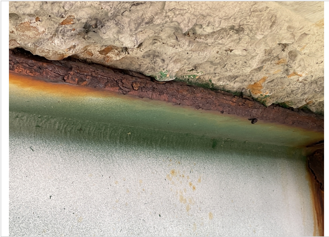
Span 3 Girder E top flange corrosion
