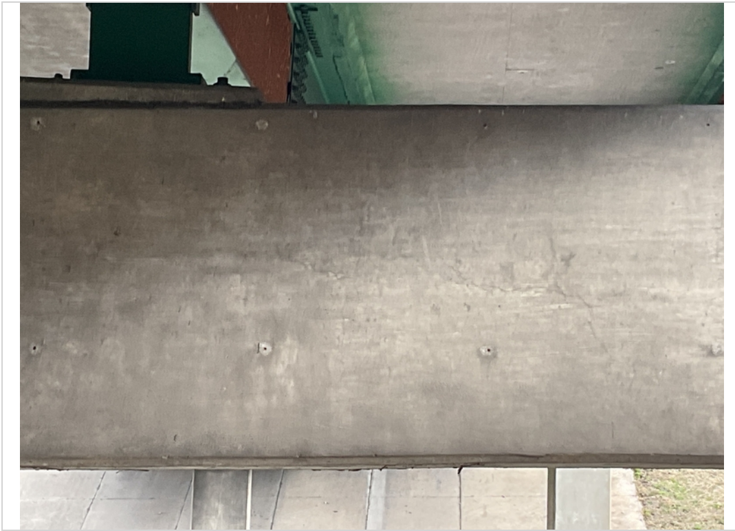
Bent 1 cap horizontal crack
