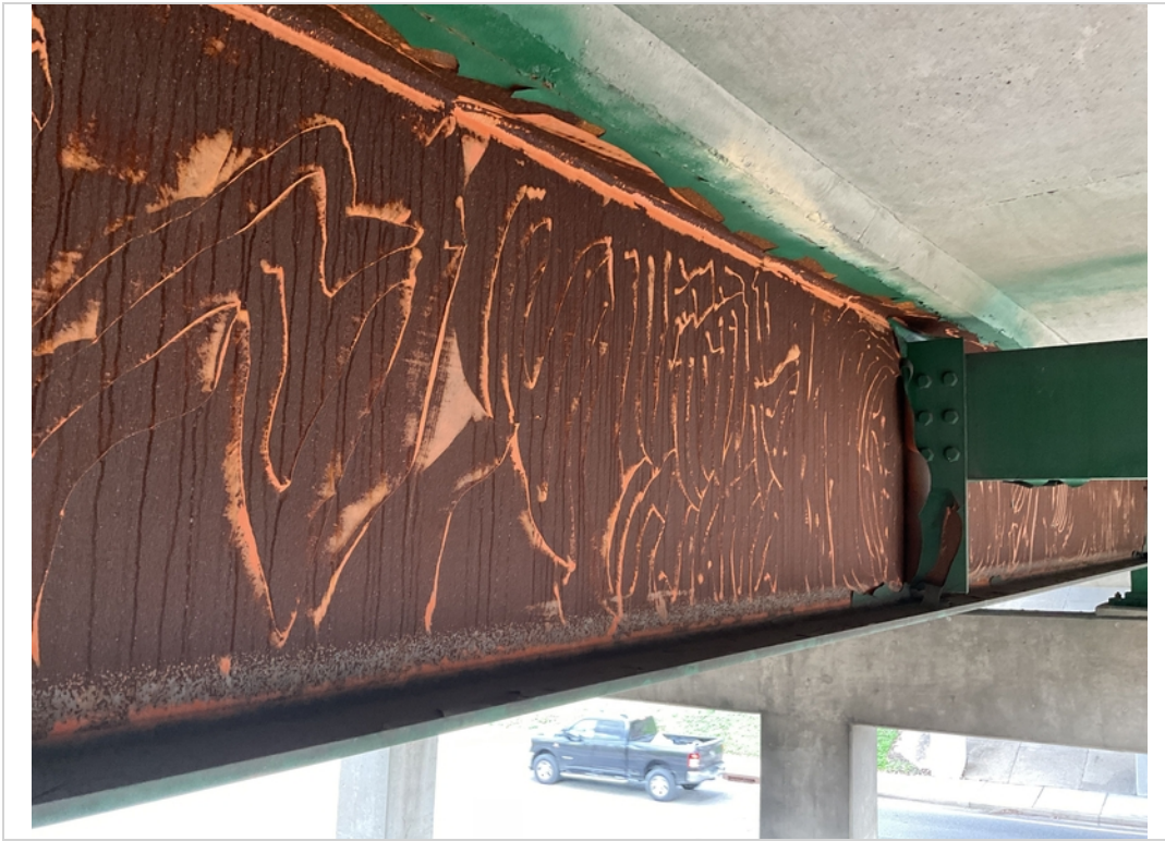
Span 1 Girder D corrosion
