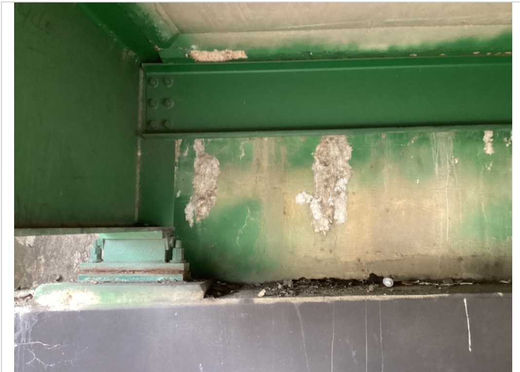
Abutment 2 backwall cracks with eff
