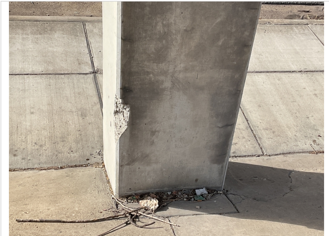
Bent 2 column B spall
