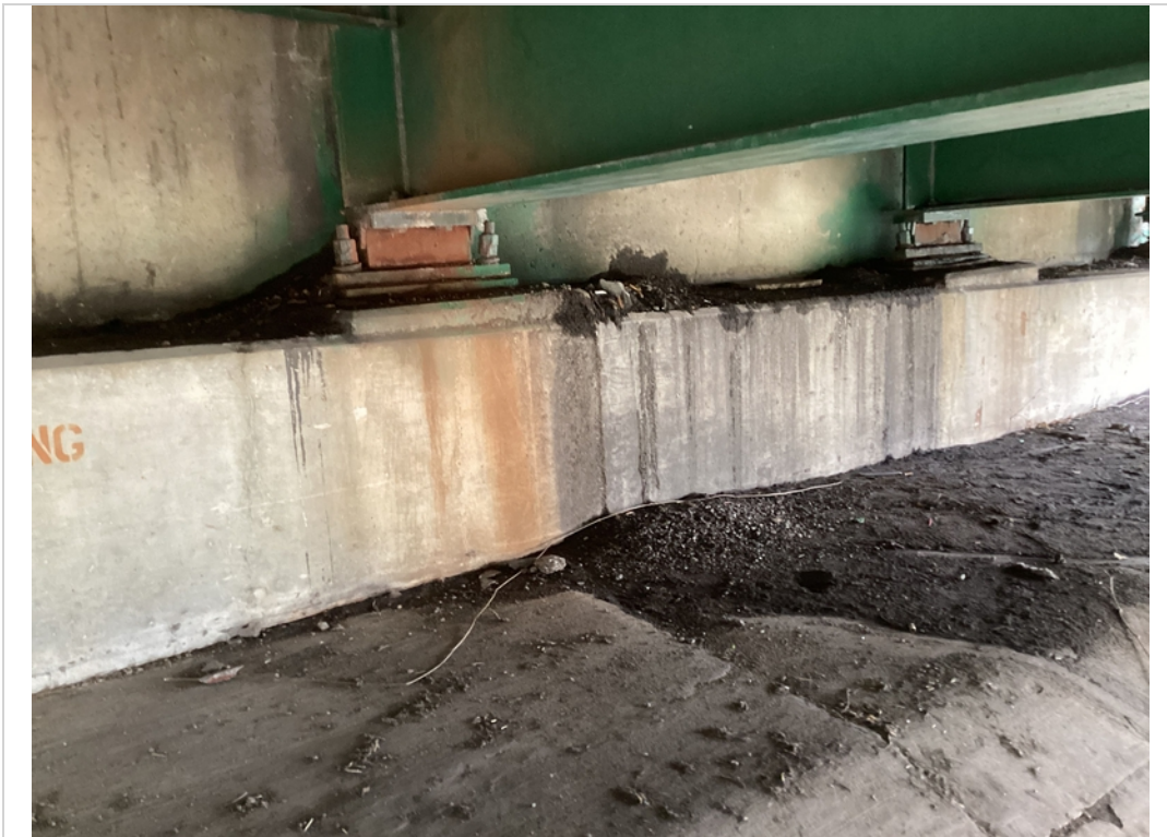
Abutment 1 water stains
