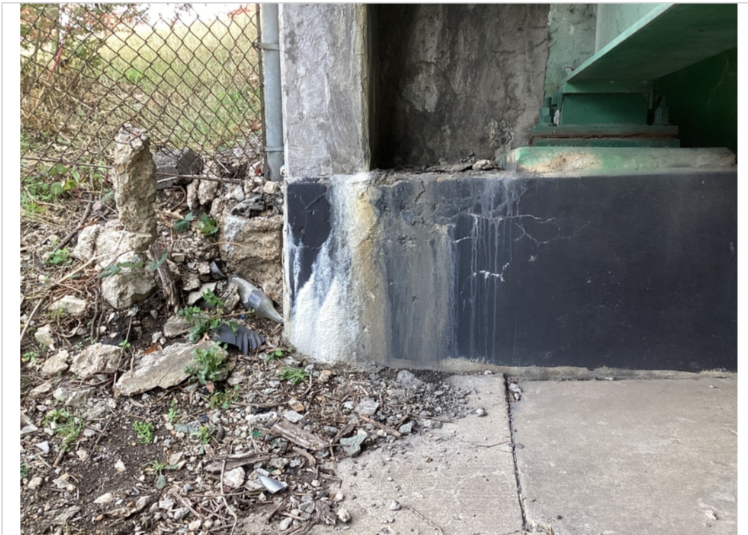
Abutment 2 cracks with eff
