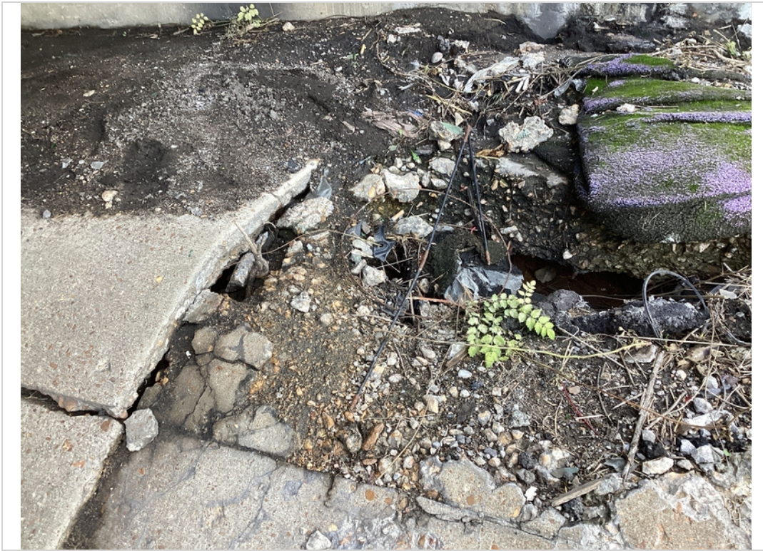
Abutment 1 slope pavement broken
