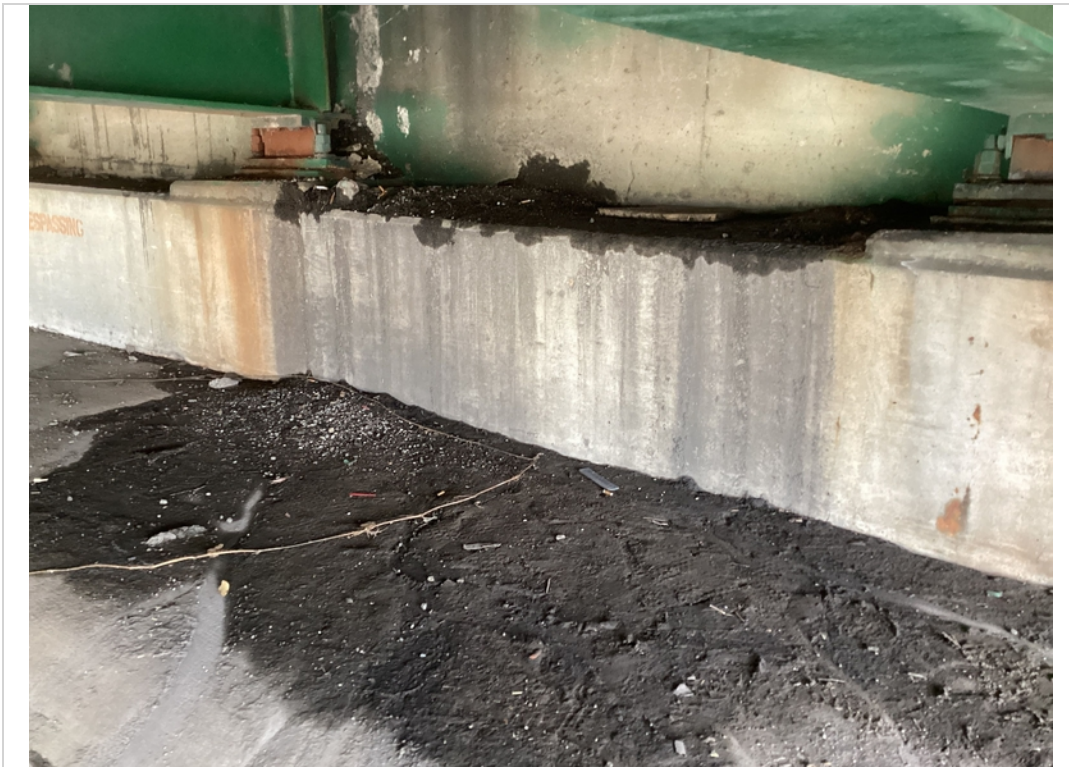
Abutment 1 debris on cap and slope pavement
