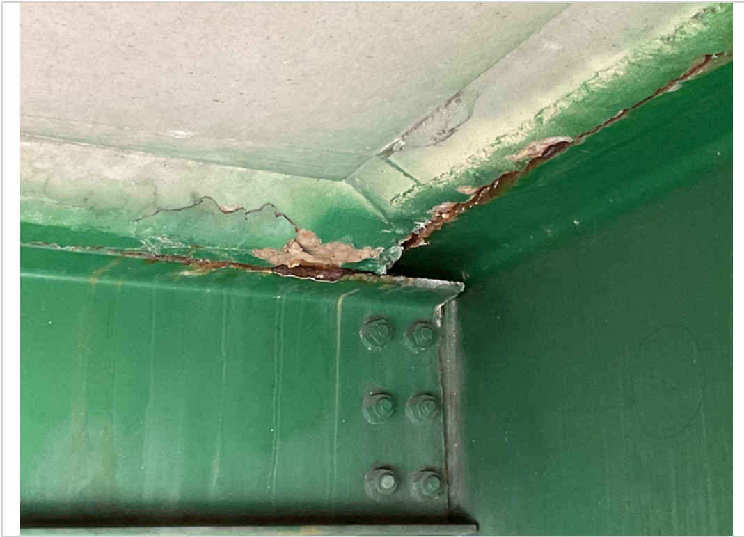
Span 3 bay C in place spall
