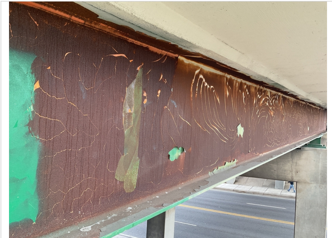
Span 1 Girder E corrosion
