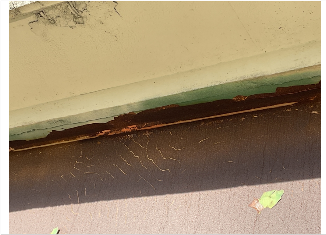
Overhang span 3 right side in place spall
