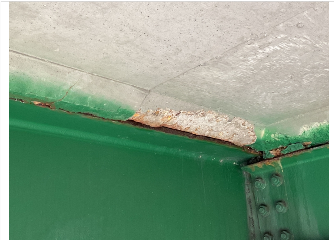
Span 3 bay D spall
