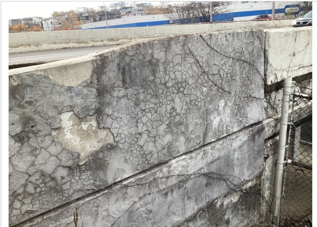
Abutment 2 left wing map cracks with eff
