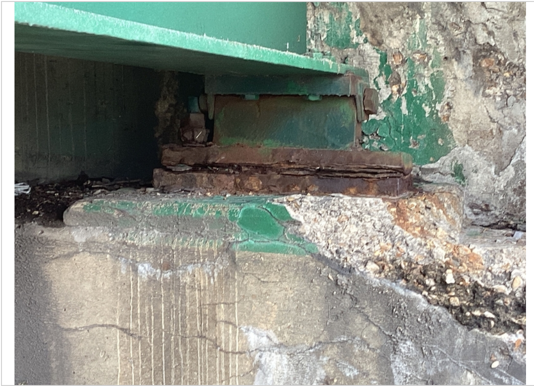
Abutment 1 bearing A heavy corrosion
