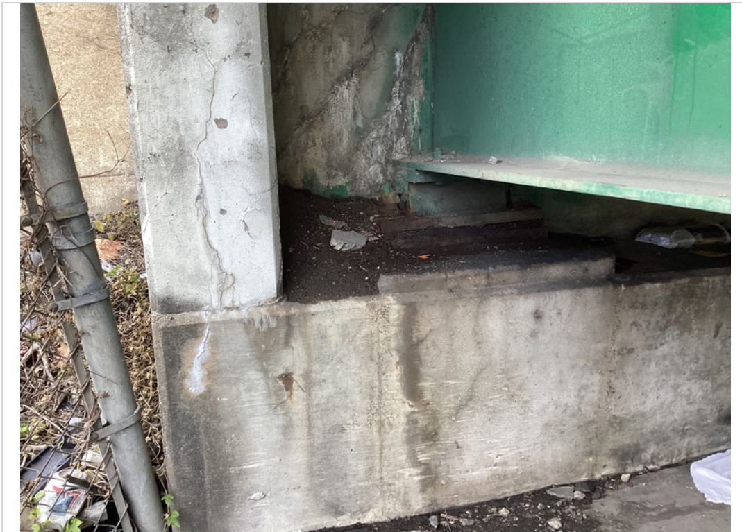
Abutment 1 bearing E rocked backstation
