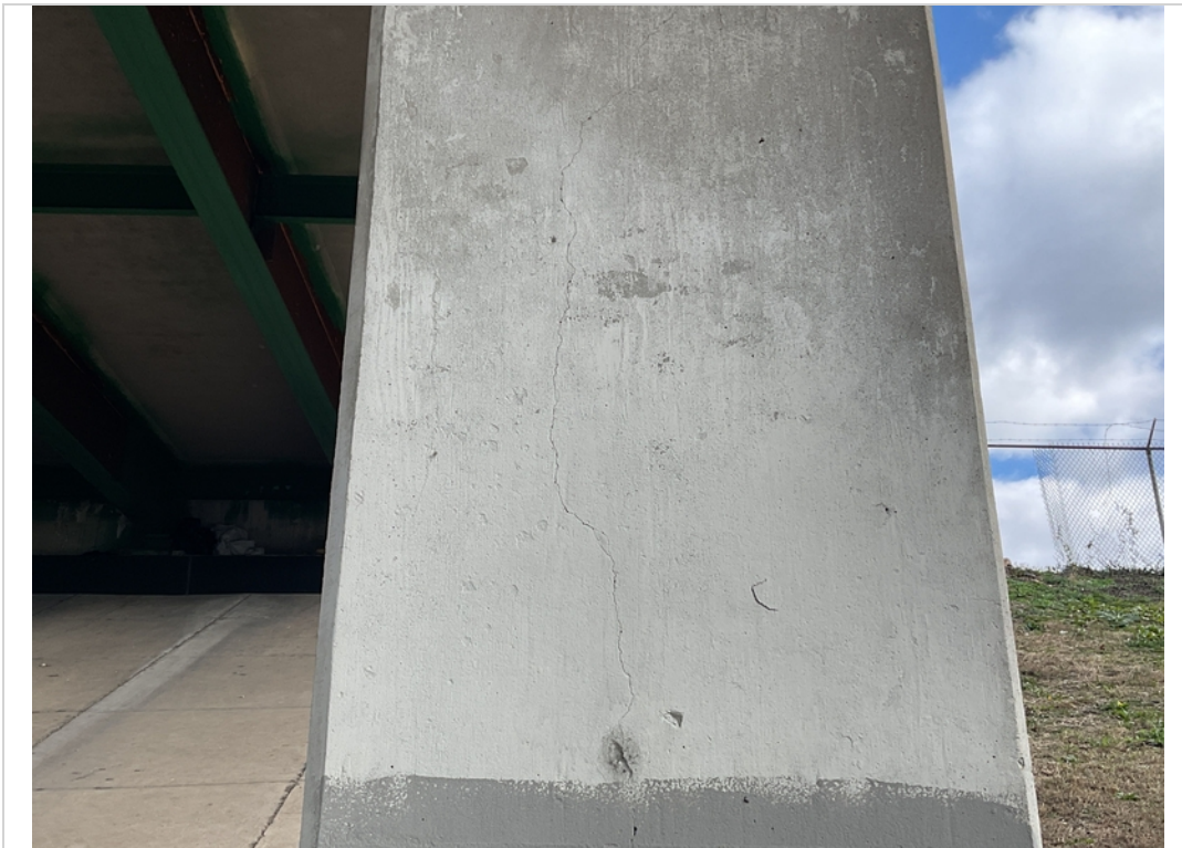
Bent 2 column C vertical crack
