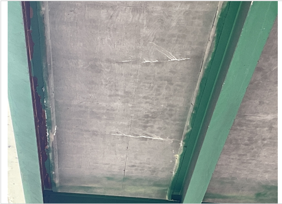
Span 2 bay A trans cracks with eff
